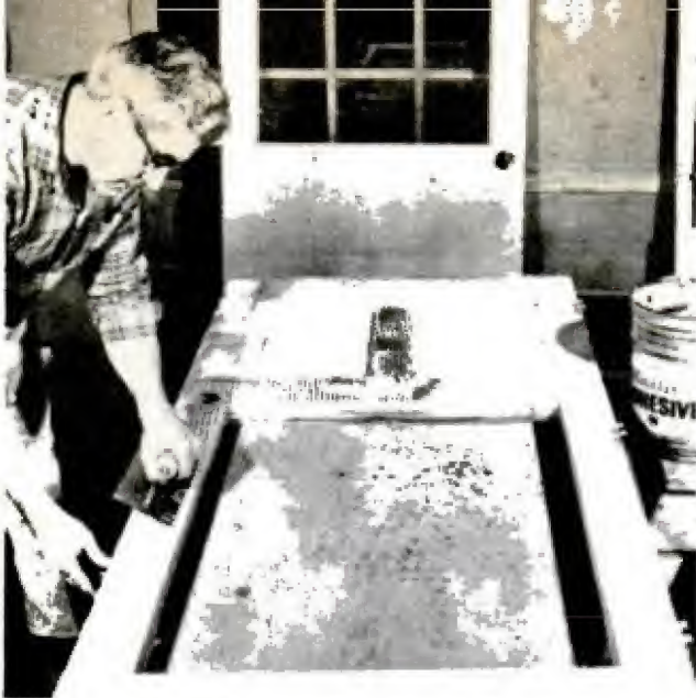
PANEL ADHESIVE simplifies facing the door interior with flush panel. Apply a thin, flat coat to door
